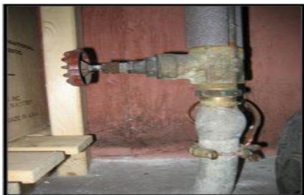
Example of Wiped Lead Joint
